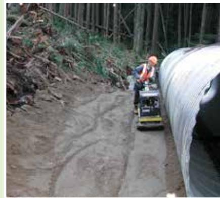
Plate compactors are common choices for the majority of the backfill envelope; jumping-jack compactors, with their smaller working area, can be maneuvered to compact under the haunches of the structure.
