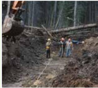
Where poor foundation soils exist, substitute suitable materials and use large aggregate for ballast, as appropriate, to improve the bearing capacity of the culvert.
