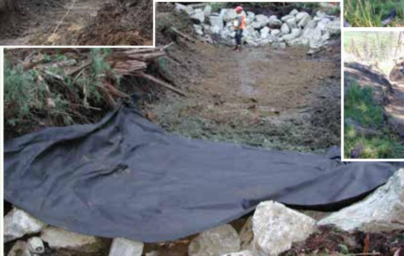
A non-woven geotextile can be placed in the culvert backfill to mitigate water piping along the outside of the culvert. In the photo to the right, an Armstrong seal has been created. The geotextile is initially placed under the culvert and then cut, spread perpendicular to the culvert barrel, and tied at the top to form a curtain in the backfill.
