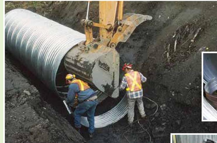
Couplers need to be secured tightly to provide a watertight seal. Gaskets can also be used with the coupler to accomplish this.
