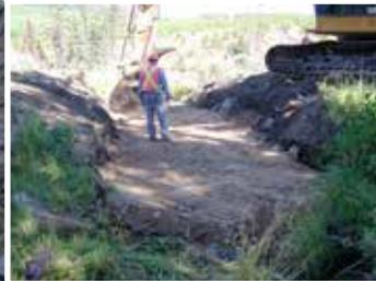
The location for the excavation was easily measured from established working points as indicated on the engineered design. The depth of excavation was measured with a construction level and rod.
