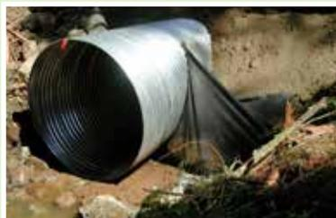
Fine granular material (e.g., sand) spread along the length of the excavation allows the culvert to be well seated into the base of the excavation.
